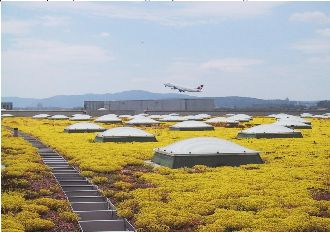
Figure 6 The Green roof in Kloten International Airport is Dock E.
